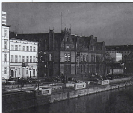
AT&T's purchase of the AT&T Telfa Network Systems Plant, top, in Bydgoszcz, below, helped win business in Poland.
