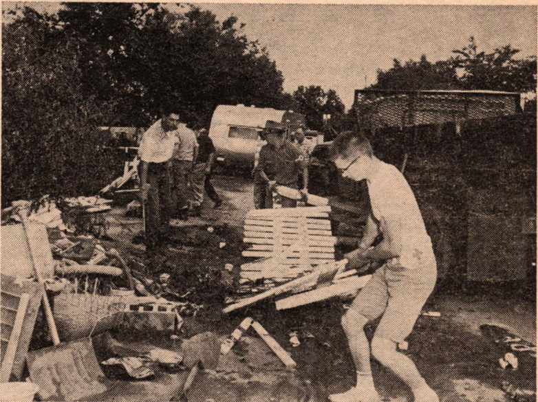
Above, Charlie Koukal, Dick Oglevie (back to camera), Claude Schade and another volunteer, wallow in mud to clean up the mess left by the devastating flood.
