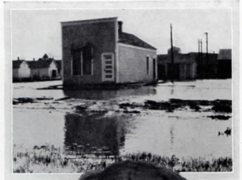
Another muddy waters scene at Philip, So. Dak. The water had receded when the picture was taken. The building is our central office.
