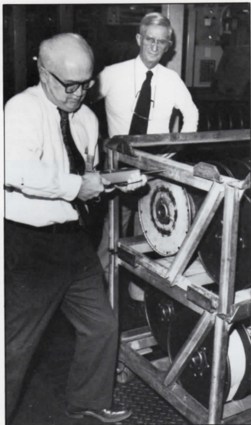
Under the watchful eyes of Dr. Lee Grant, 140, Dan Boland, 524, measures the force required to start wheeled pallets at PIC tandem lines.
