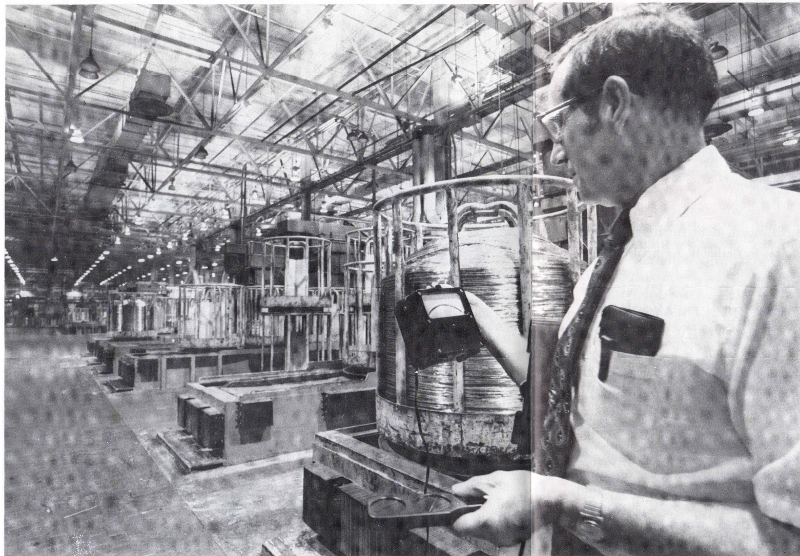
At the Atlanta Works, Don Timmerman checks the light level of new energy-efficient high-pressure sodium lamps. The new lamps will save about 2,200,000 kilowatt hours of energy and $91,000 per year.
