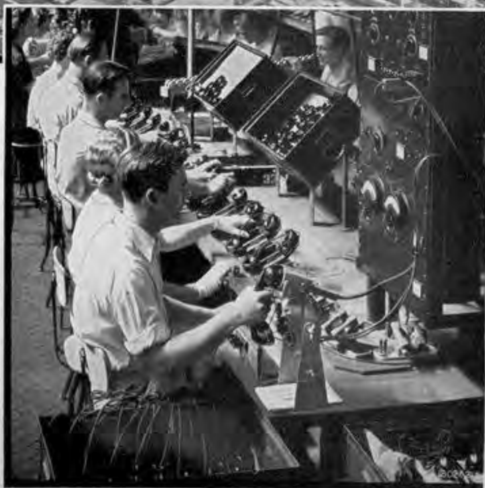
Every telephone must pass an electrical voice test.
