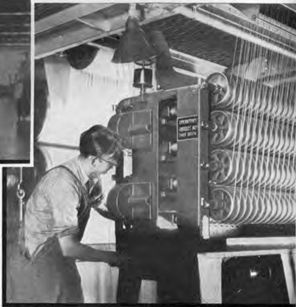
Makes paper insulation on 60 wires at once.
