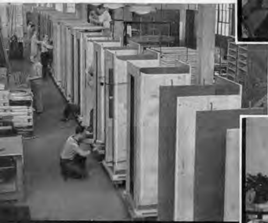
Booths speedily built on the assembly line at the Queensboro Works.
