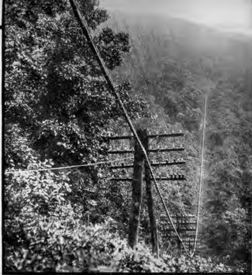
A vast network of wire and cable traversing the nation from coast to coast, overhead...
