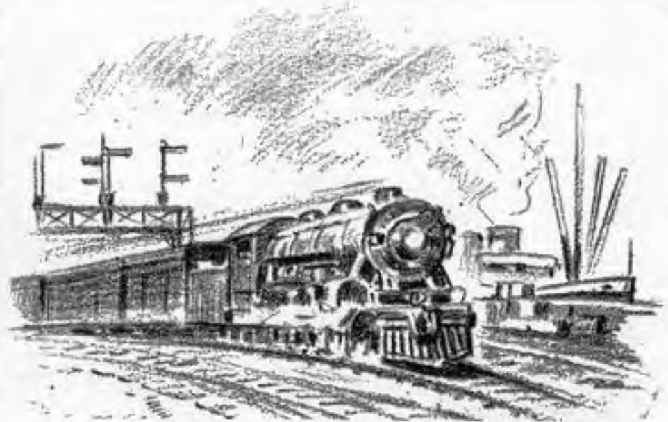
By railroad, ship and air, telephone supplies flow in a never ending stream.
