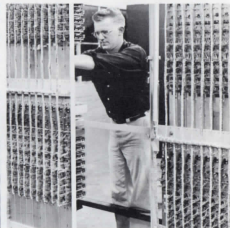
Merle Giddings, W. E. installer, checks numbers on terminal strips on block relay frame made in the Omaha Shops for hometown telephone service.
