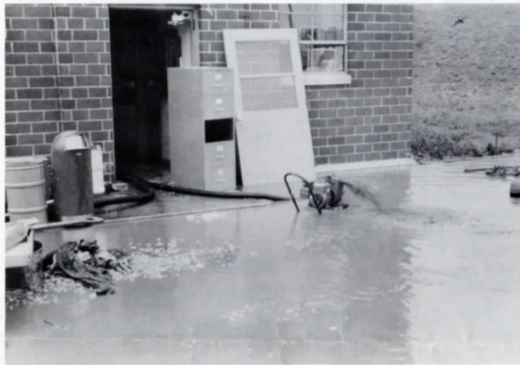
Sewage disposal plant building was flooded and had to be pumped out.
