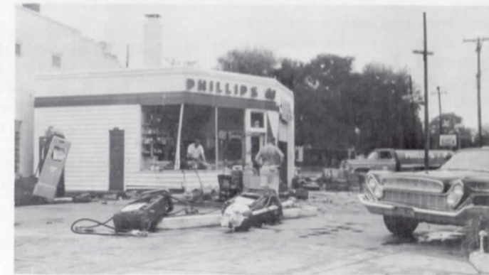
Gasoline pumps at a Papillion station were knocked down like ten-pins by the water.
