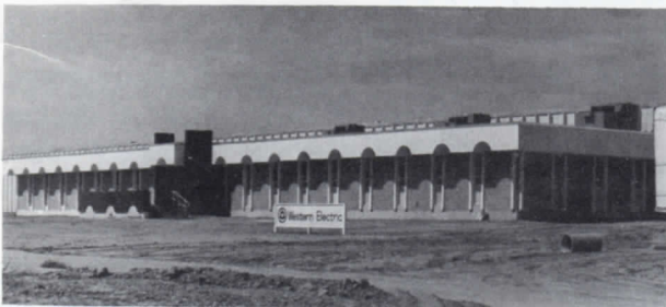
Building 613 takes on a new clean styling as construction proceeds.
