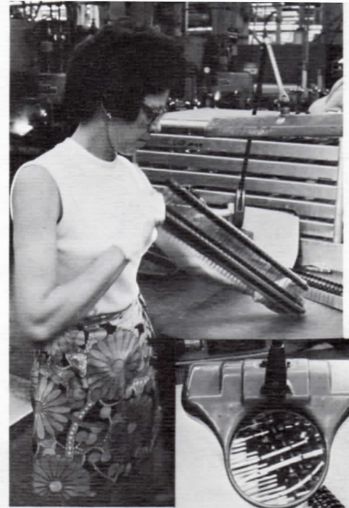
Wire blocks which have been formed, clipped, and had contacts welded to each wire end are unloaded and checked by Exit Operator, Betty Snodgrass (above).
