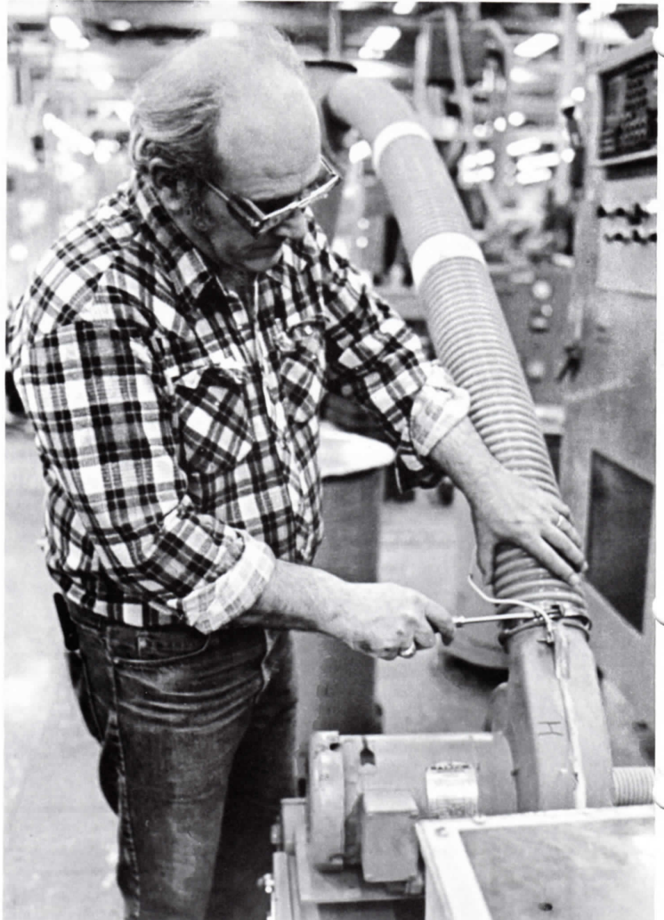
BETTER HOSES . . . Dept. 425 machine setter Ron Hallett adjusts one of the new hoses on the regrind barrels that have been installed to prevent plastic particles from escaping. Ron is leader for Quality Circle No. 2.
