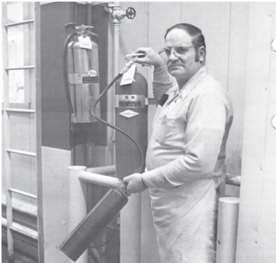
THE RIGHT CHOICE . . . Floor hand Larry Tremayne of Dept. 235 holds a Type BC fire extinguisher used for chemical and electrical fires. A Type A water extinguisher is mounted beside him.
