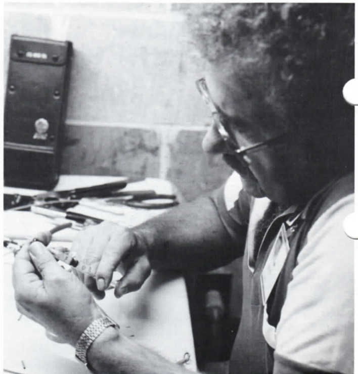
INSTALLATION . . . Jody Brewer of Dept. 269 (left) helped out in the Works' data center by wiring 110 patch panels that interface with the fiber optic backbone of the local area network. Below left, an installer cuts glass fiber at the terminating end and Bill Reisz (below right) uses a syringe to inject epoxy glue into a connector to hold the glass fiber in place prior to termination. Reisz pulls fiber optic cable (opposite page) through conduit at a junction box located in Building 30.
