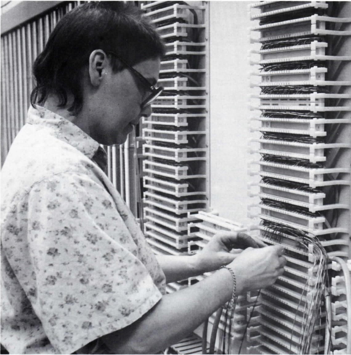
INSTALLATION . . . Jody Brewer of Dept. 269 (left) helped out in the Works' data center by wiring 110 patch panels that interface with the fiber optic backbone of the local area network. Below left, an installer cuts glass fiber at the terminating end and Bill Reisz (below right) uses a syringe to inject epoxy glue into a connector to hold the glass fiber in place prior to termination. Reisz pulls fiber optic cable (opposite page) through conduit at a junction box located in Building 30.
